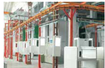
In house Powder Coating Facility for Canopy
